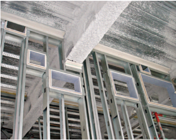
Figure 10 Prepared openings in a drylined partition (note spacings between openings may differ)
